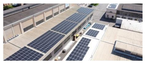
of 961 photovoltaic modules were initially installed – which is equivalent to an area covering 1,634 m<sup>2</sup> – on the roofs of the office and production buildings at its Austrian facility. 43% of the power that Bekum uses every
